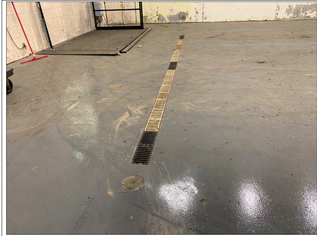
Photo 9: Trench drain in food waste room on southwest corner of building.
