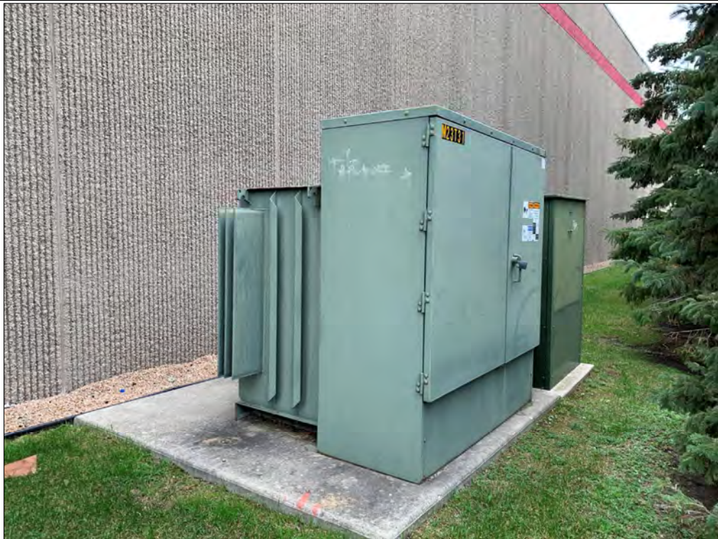
Photo 6: Pad-mounted transformer on north side of building.
