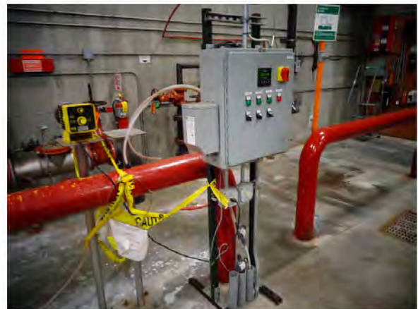
12. wastewater agitation tank controls
