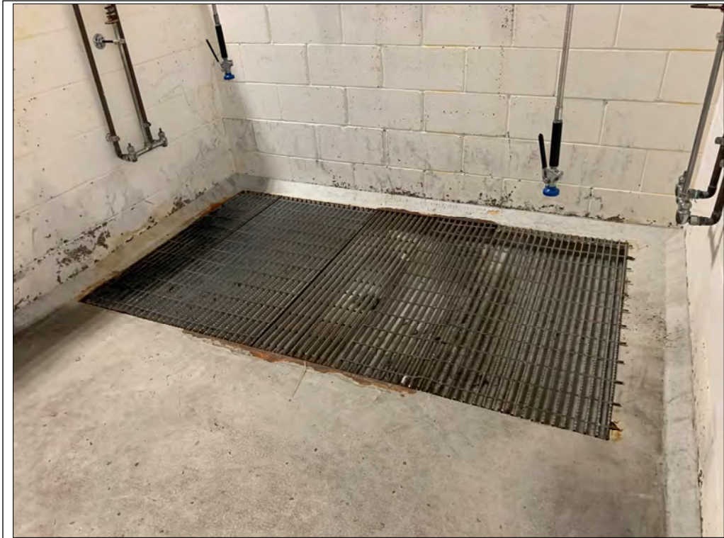
Photo 13: Large drain in employee prep area.
