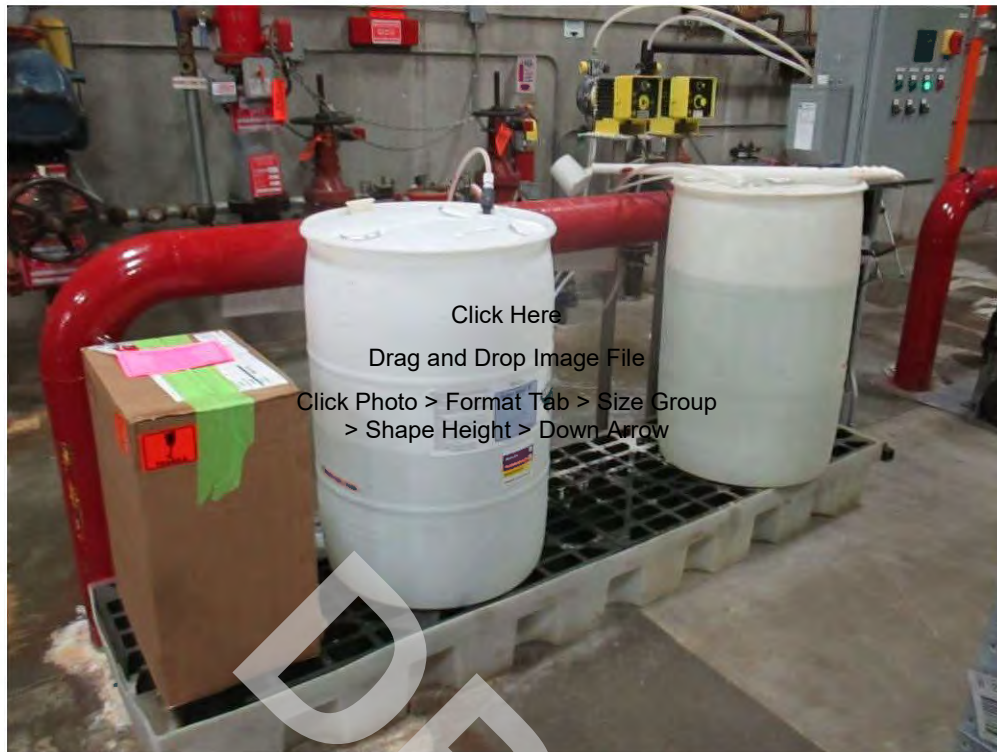
Photo 3: Wastewater treatment chemicals on secondary containment
