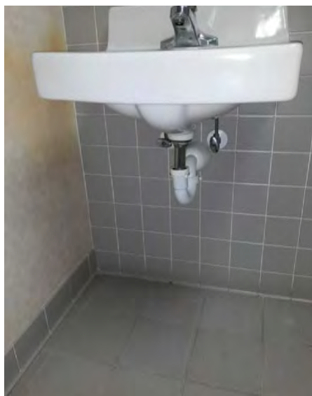
Office Restroom Sink Drain Pipe
