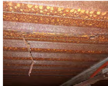
Rusted Bar Joist
