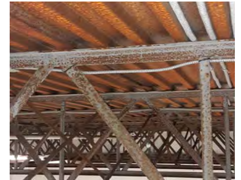
Rusted Bar Joist
