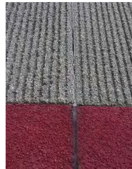
Exterior Wall Panel Sealant
