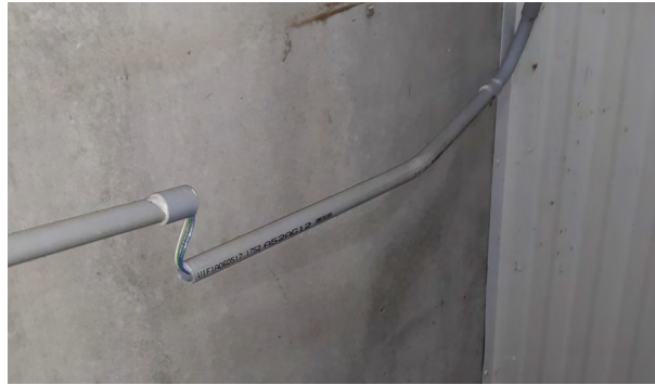
Exposed Wires
