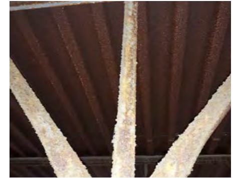
Rusted Bar Joist
