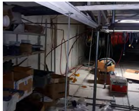
Suspended Ceiling Supports
