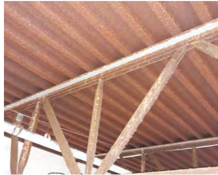
Rusted Bar Joist
