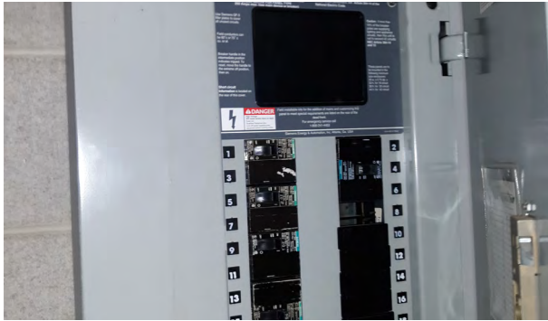
Missing Breaker Cover
