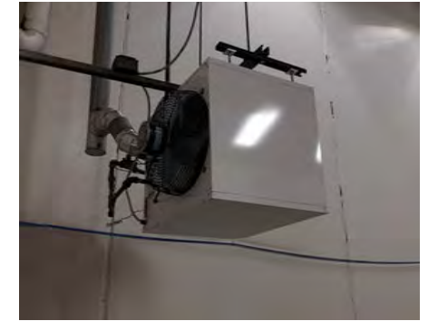
Ceiling Mounted Heaters
