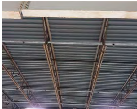
Rusted Bar Joist
