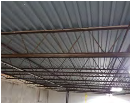
Rusted Bar Joist
