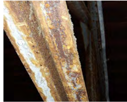
Rusted Bar Joist
