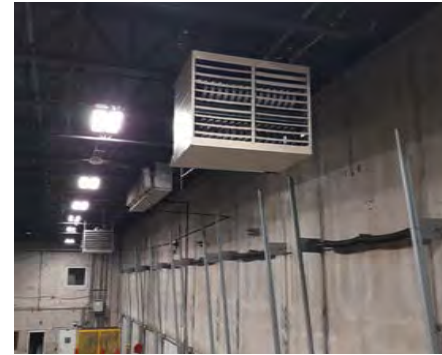
Ceiling Mounted Heaters
