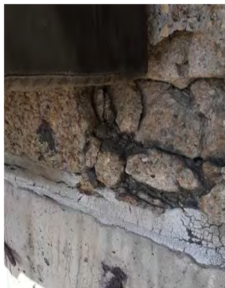
Precast Wall Damage
