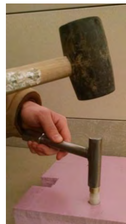
Photograph 6: Installation Tool w/ Mallet
