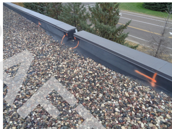
40. Section of EPDM roofing pulling away from parapet.
