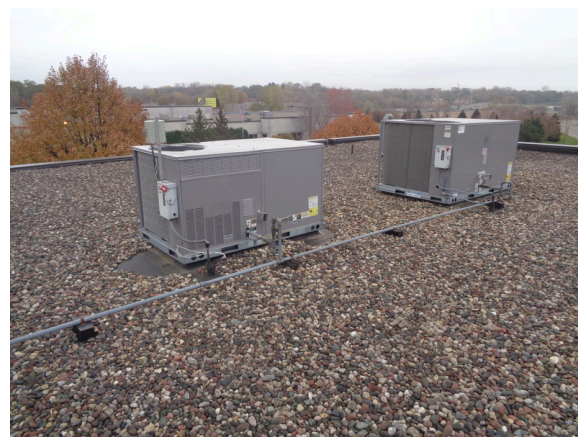
42. Rooftop mounted packaged HVAC units.
