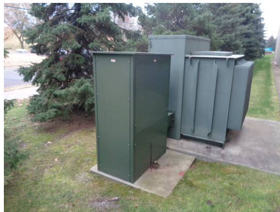
50. Pad mounted electric transformer north of the building.
