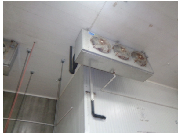
44. Typical cooling unit in refrigerated area.
