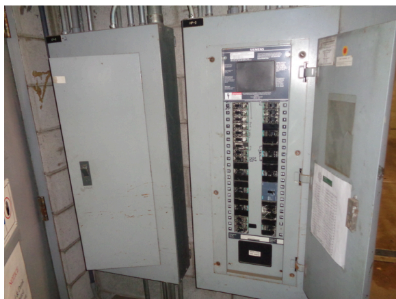
53. Electric subpanel in tenant space.
