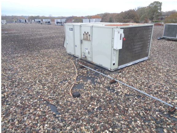
43. Original rooftop packaged HVAC unit.
