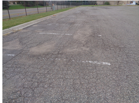
14. Asphalt pavement with alligator cracking, east side of parking area.
