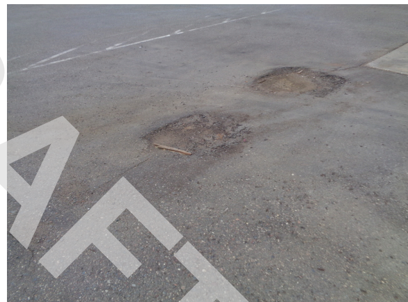
16. Damaged section of asphalt pavement at loading dock.
