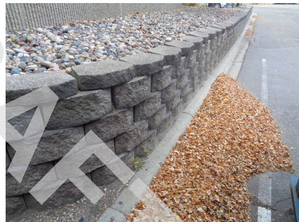
22. CMU retaining wall adjacent to entrance with slight bow.
