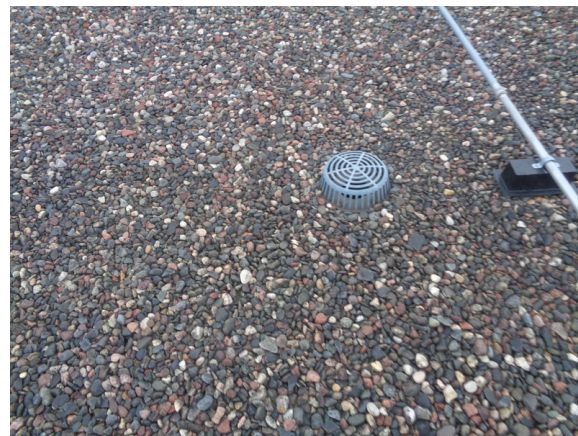
38. Interior roof drain.
