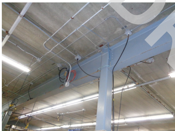
27. Structural steel support and precast concrete panels.
