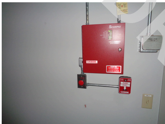
57. FM-200 fire system for server room.
