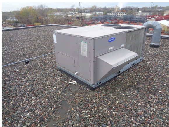
41. Rooftop mounted packaged HVAC unit.
