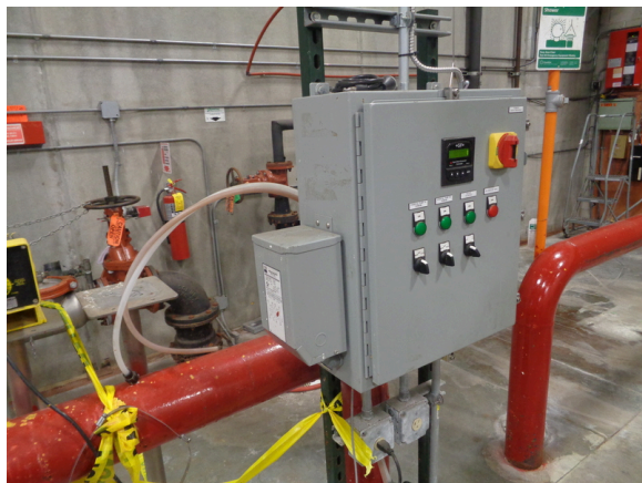
49. Waste water agitation tank controls.
