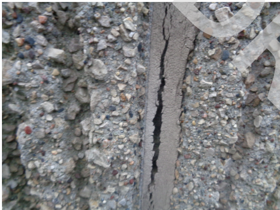
33. Cracked sealant at tilt-up concrete panel.
