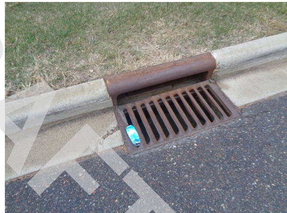
10. Concrete catch basin on west side of Site.
