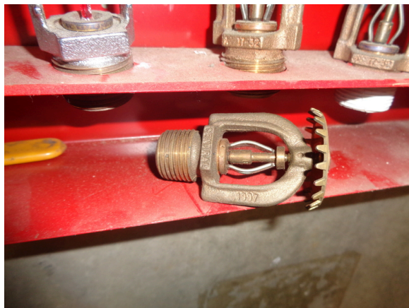
55. Central brand sprinkler head from 1997.
