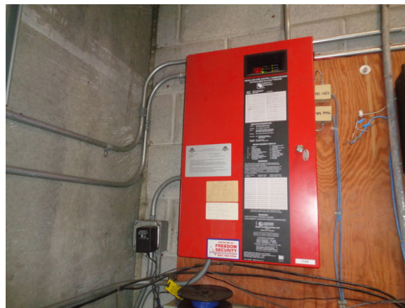
56. Fire alarm control panel.
