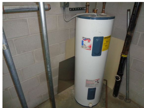
48. Electric water heater for restrooms.
