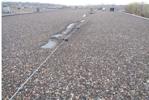
37. Overview of west addition ballasted EPDM roof.
