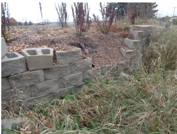
23. Damaged section of CMU retaining wall, southwest corner of Site.
