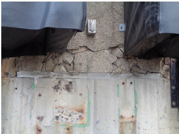
35. Damaged section of precast concrete at loading dock.
