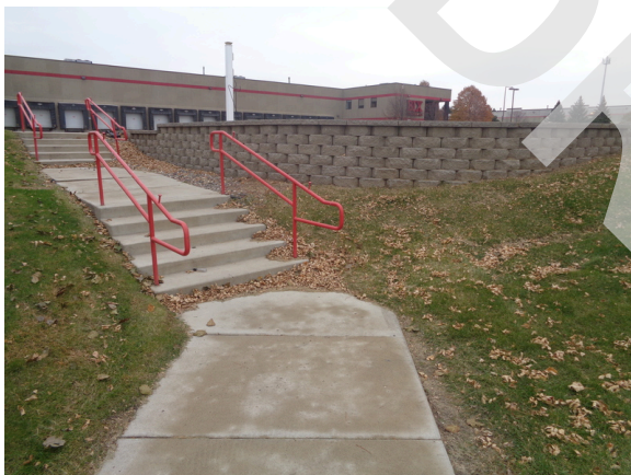
21. CMU retaining wall and concrete stairs at south side of Site.
