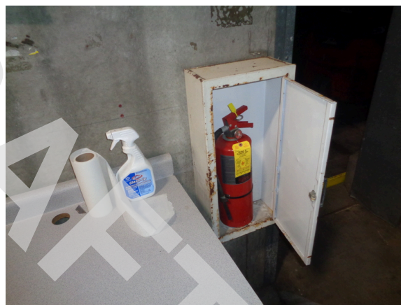
58. Fire extinguisher with expired tag.
