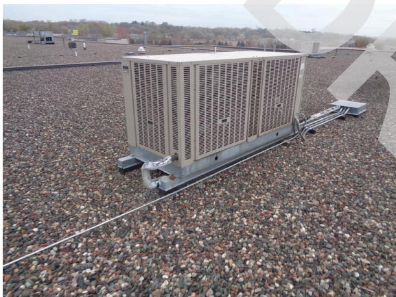
45. Cooling unit roof mounted condenser.
