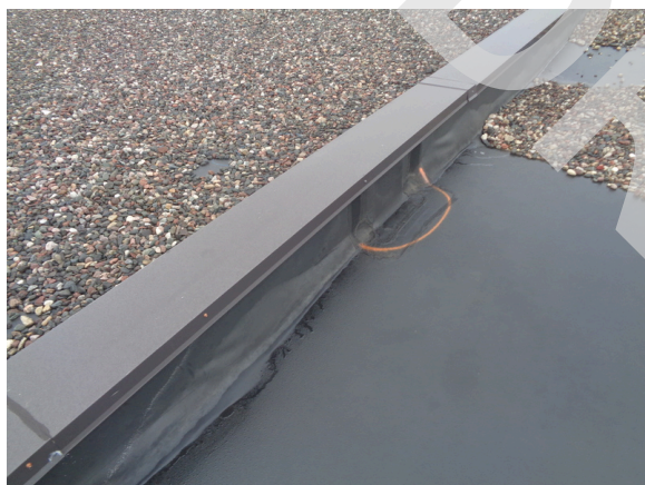
39. EPDM roofing pulling away from parapet.
