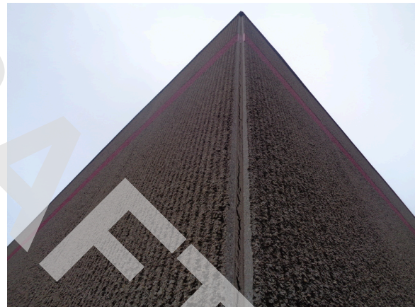
34. Cracked caulking at the northeast corner.
