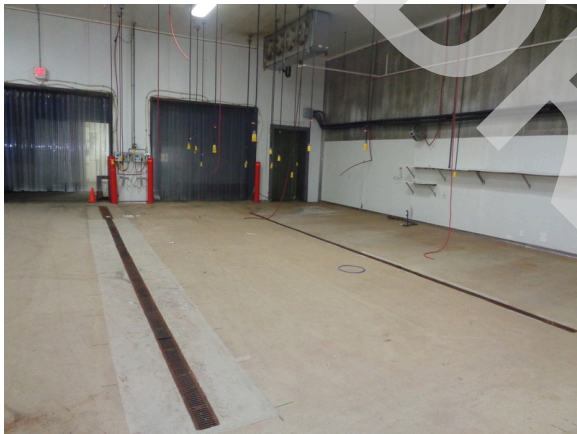
69. Floor drains in refrigerated warehouse.
