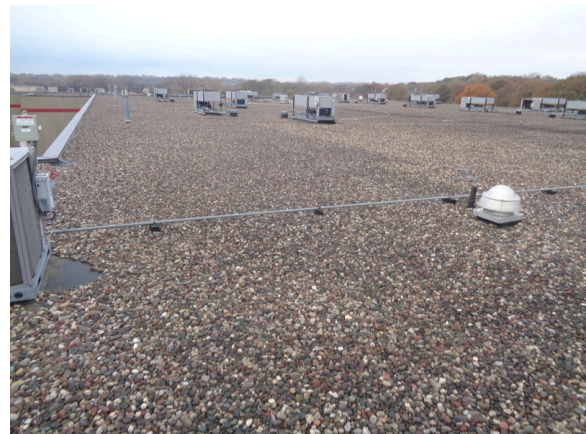
36. Overview of ballasted EPDM main roof.
