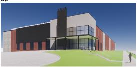
iv. Third example – simplifies the vestibule and pushes it inside of the building, maintaining more prominent glazing around the corner, transpired solar collector wraps around the corner (takes solar energy and helps to heat the building)
